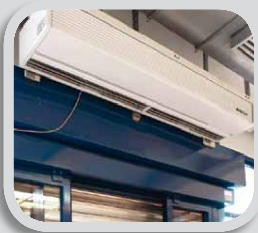
Fig. 1 - The traditional and cumbersome air barrier mounted separately to the door
